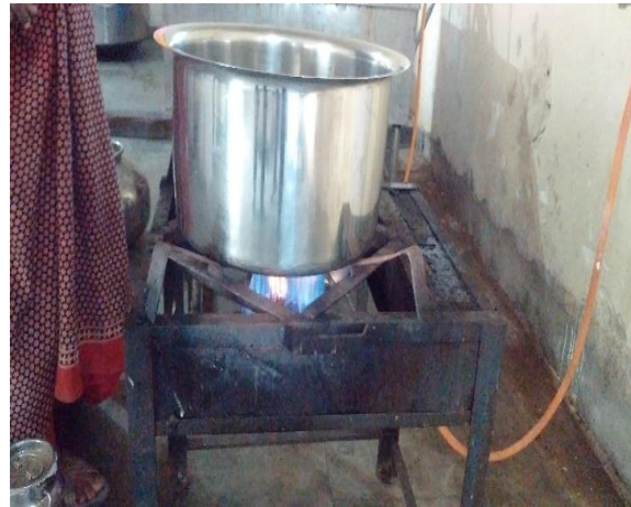
Bio Gas Flame in Kitchen with fitments
