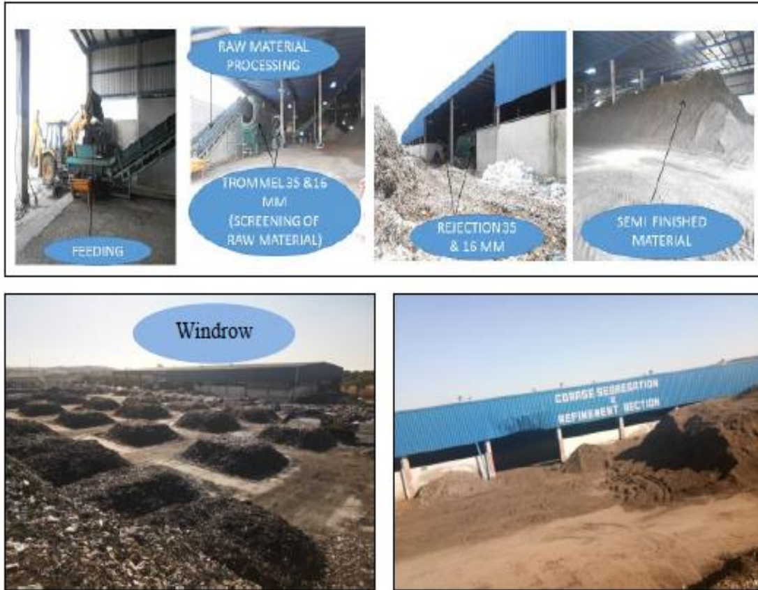
Figure 5: IL & FS Composting Plant at Sewapura (Jaipur)
